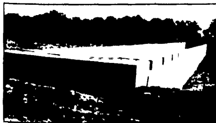
300' Long Manure Pit For Hog Confinement
