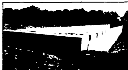
300' Long Manure Pit For Hog Confinement
