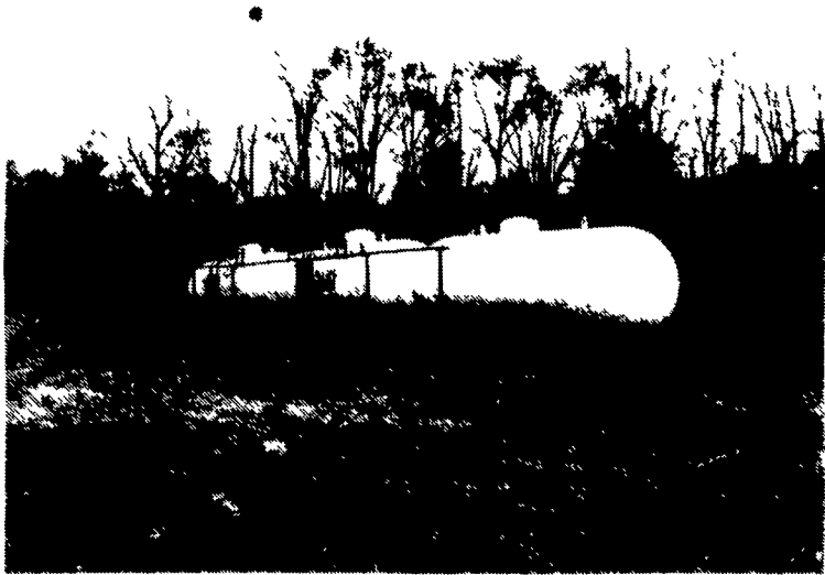
Of the three propane tanks located at the rear of the veal raising facility, two are dedicated to fuel two forced-air heaters, while the nearest tank is reserved to serve a large backup generator.
