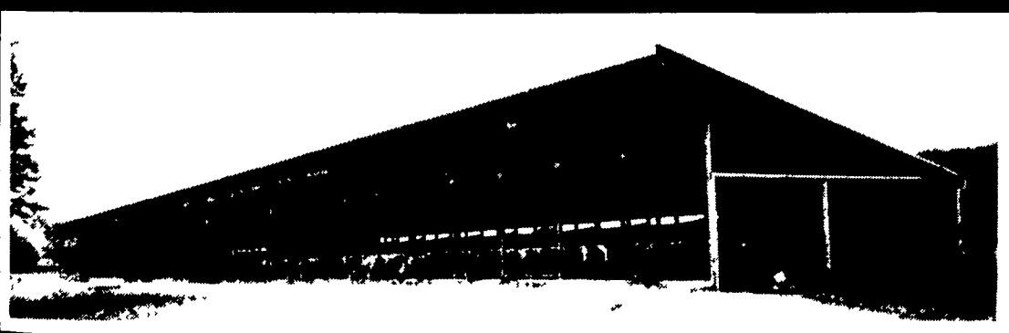
New 332' Heifer Facility Featuring 8' Deep x 12' Wide Manure Storage System With Waffle Slats
