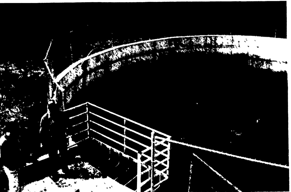
A heavy rain works on the manure in the lot, but is funneled through a concrete thruway into this 200,000-gallon capacity circular in-ground concrete storage structure. The structure, installed in 1991, is emptied twice a year, according to Dave Becker, right.
