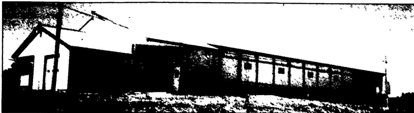
40'x140' Milking Facility
