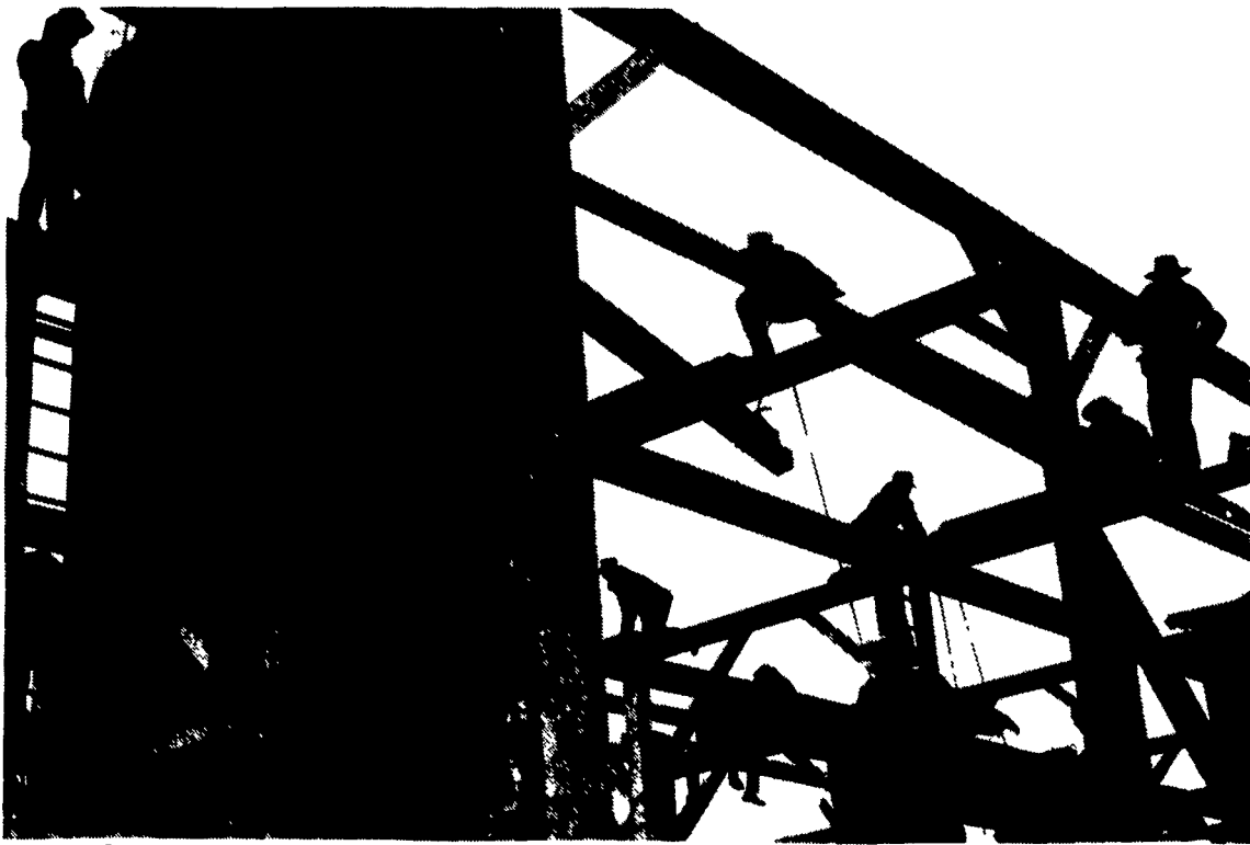
At the call of the construction foreman supervising from the floor below, a main beam running the length of the barn gets hoisted up into place.
