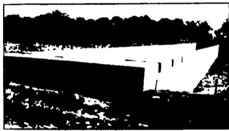
300' Long Manure Pit For Hog Confinement
