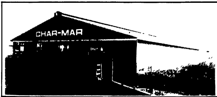
80'x300' Free Stall Building Built In Maryland
