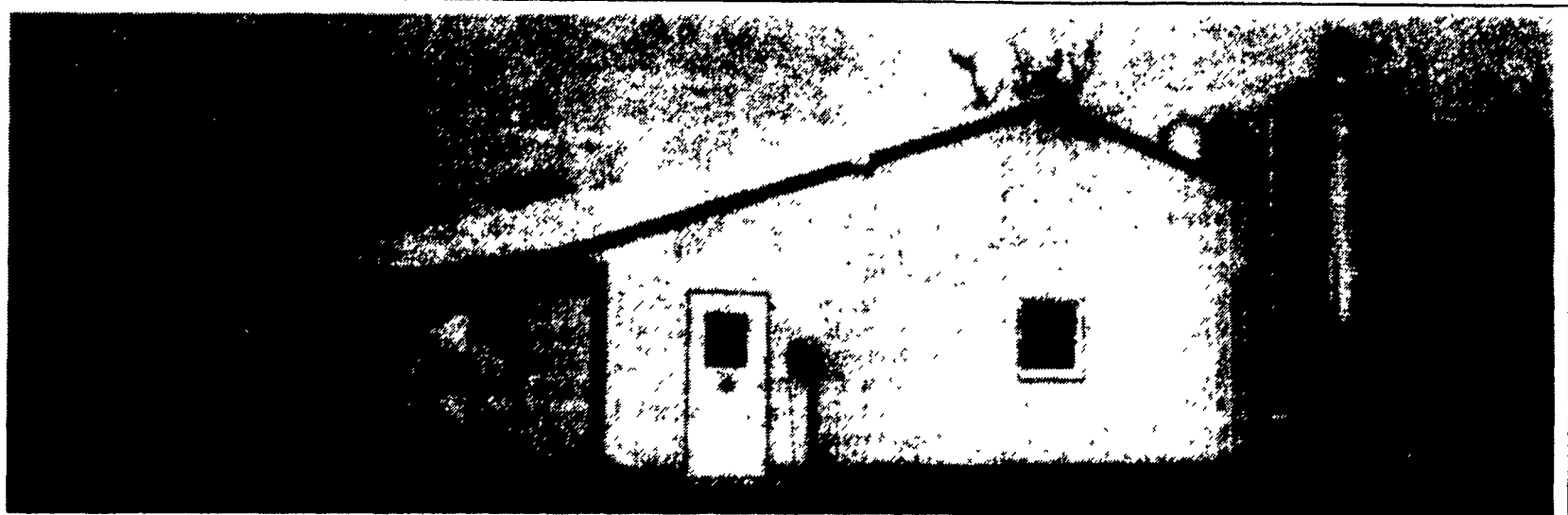
37'x116' Farrowing And Nursery Barn With CHORE-TIME Bins And CHORE-TIME Flex Auger Fill Systems
