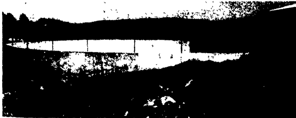
12' x 83' Diameter Circular Manure Storage
