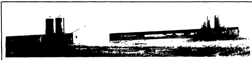
This 2-stage facility features a 50'x 215' brooder building and a 50'x 520' growout building designed for 8,000 Toms.
