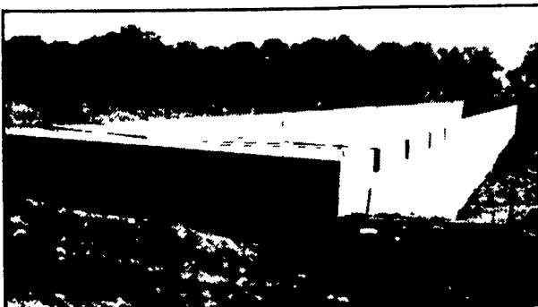
300' Long Manure Pit For Hog Confinement
