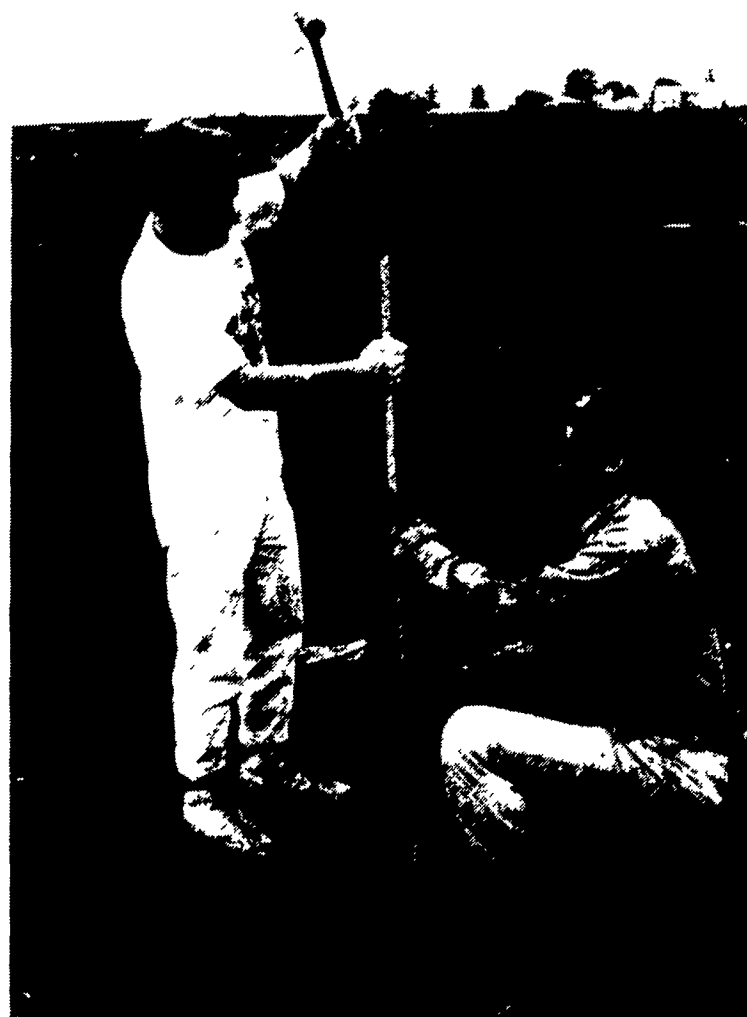
Omer Brubaker, SCS, right holds up recycled plastic posts while Terry Worall hammers them in.
