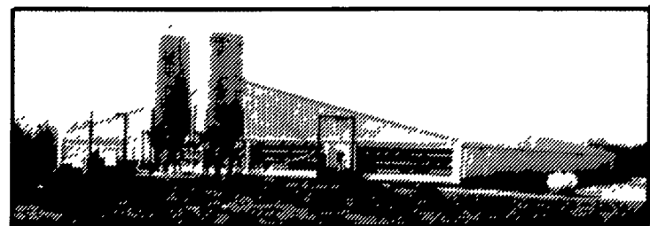
101'x245' 3000 head tunnel ventilated hog finishing house
