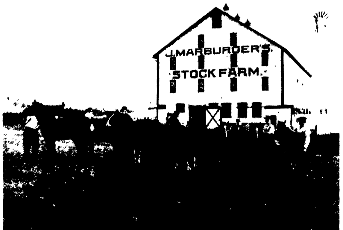
This beautiful landmark bank barn on the Marburger Farm Dairy was destroyed by fire in 1979. The historic structure measured 88 feet wide, 138 feet long, and 52 feet high. It contained four barn floors large enough to circle wagons.
