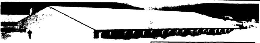
The FIRST Multiple Room **Cross Tunnel Ventilated 5 Room** Finishing Building: 125'x203' With Individual Deep Pits
