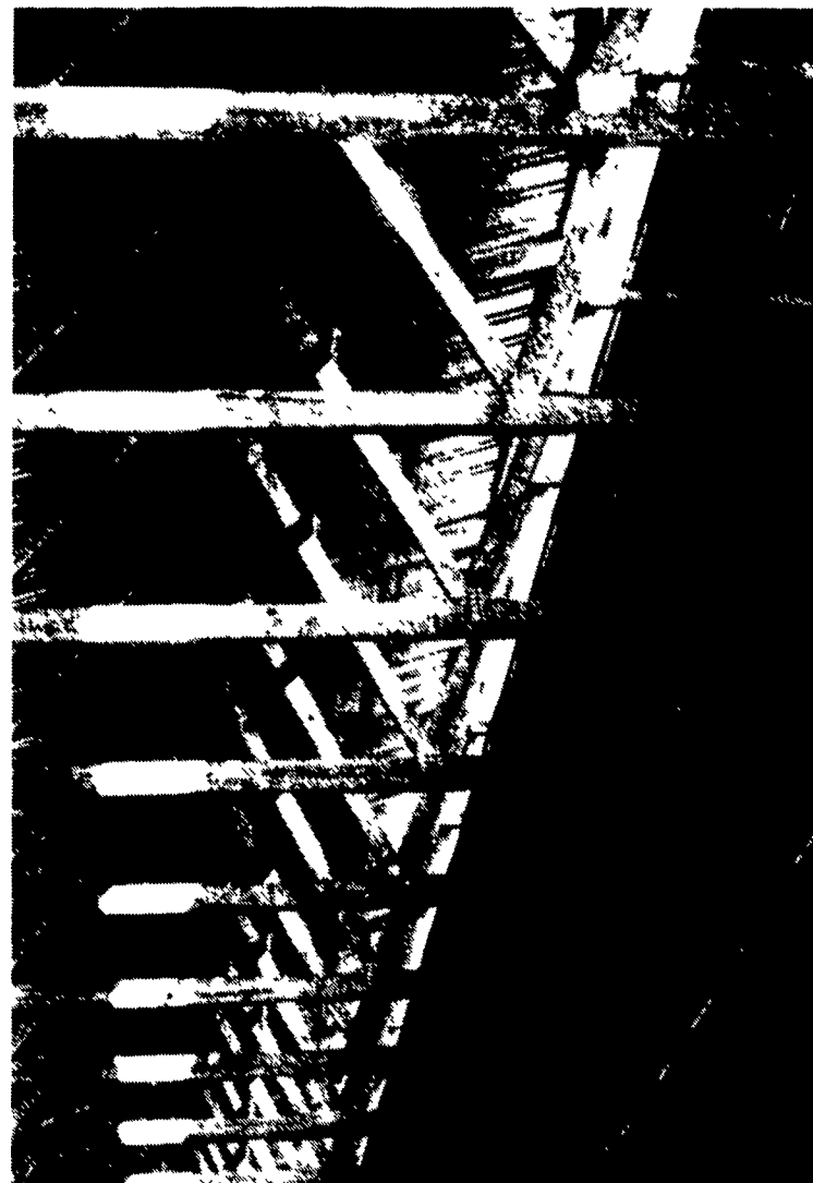
Looking up from the floor of the new Hershey brothers' freestall building, the unique roof structure is apparent. Sunlight comes through the open roof peak, casting light on rafter beams. Interior, suspended rainspouting is the flat, four-tracked sheet going from the top right of the picture to the bottom middle.
