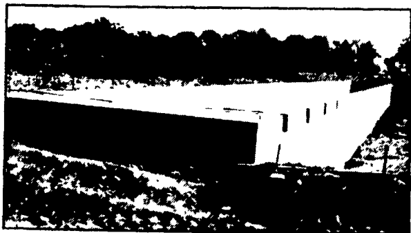
300' Long Manure Pit For Hog Confinement
