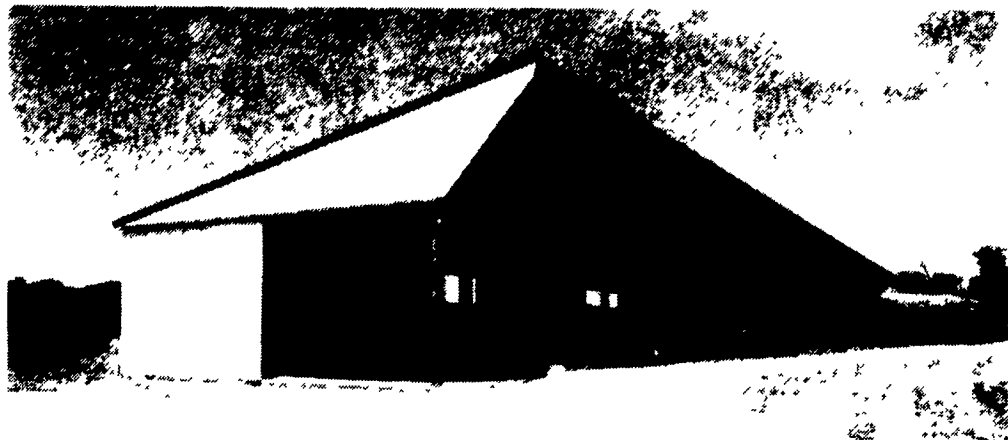
Virginia Style Heifer Barn With 8' Deep, 180' Long, 12' Wide Slatted SCS Approved Concrete Manure Pit
