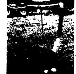
11/2" dia. delivery tubes drop foam at ground level.
