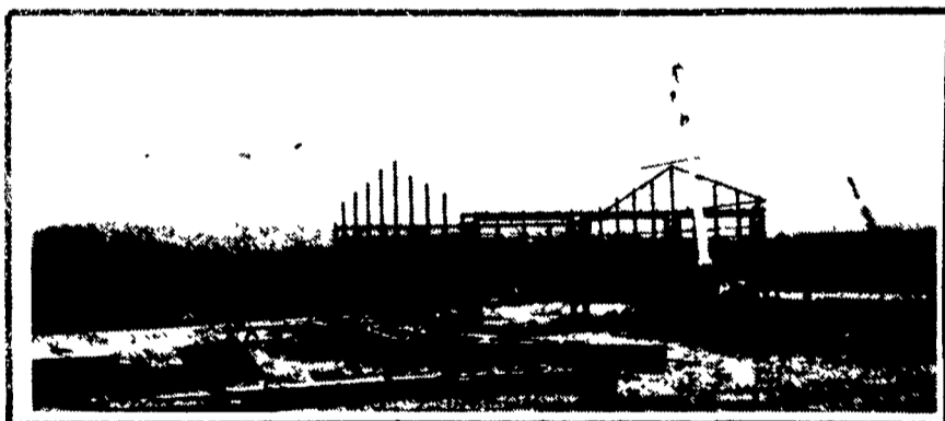
Post frame Building Package: Lumber, Steel Cladding, Engineered trusses, Glu-Lam Posts & Glu-Lam Beams.
