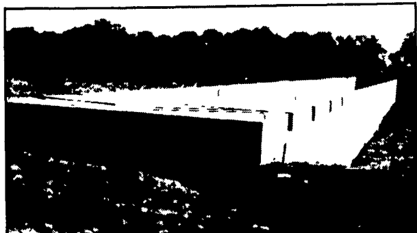
300' Long Manure Pit For Hog Confinement
