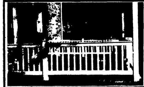
PVC Railing & Resource Lumber Deck
