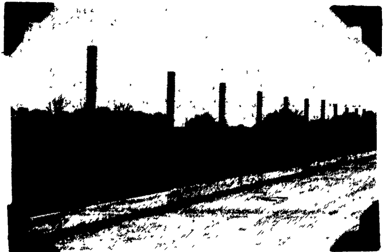
When Hershey started construction, the posts went up first.
