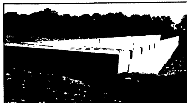
300' Long Manure Pit For Hog Confinement
