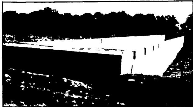
300' Long Manure Pit For Hog Confinement
