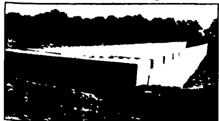
300' Long Manure Pit For Hog Confinement
