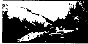
92' Boom Placing Concrete
