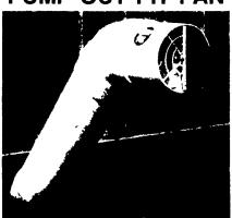
Many manure storage pits have been constructed without providing for ventilation of the pit, particularly in buildings constructed several years ago when pit storage was first popular
