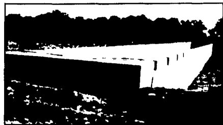
300' Long Manure Pit For Hog Confinement
