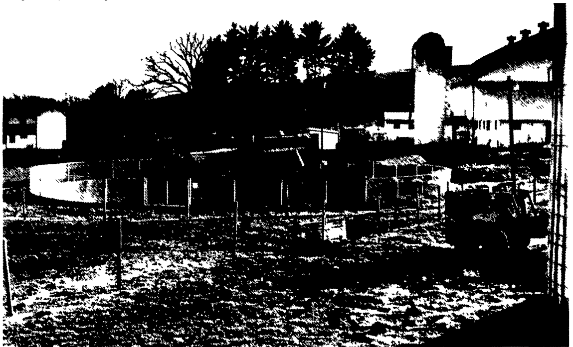
New manure storage system recently installed.
