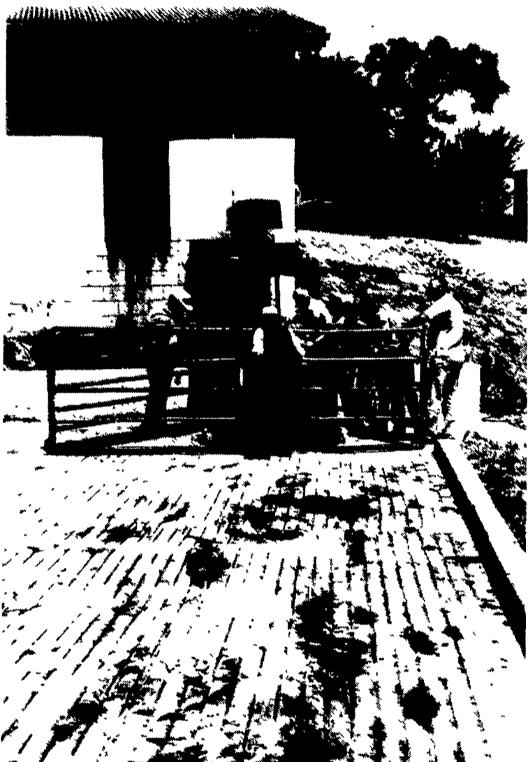
Several farmers peer down into a manhole like opening at the Jay Brandt farm in Bachmanville. The gutter scraper is visible above their heads. The grooved cement in the foreground drains a heifer yard not seen to the left, and keeps all manure and manure contaminated drainage from going anywhere else but down the manhole, like a huge french drain.
