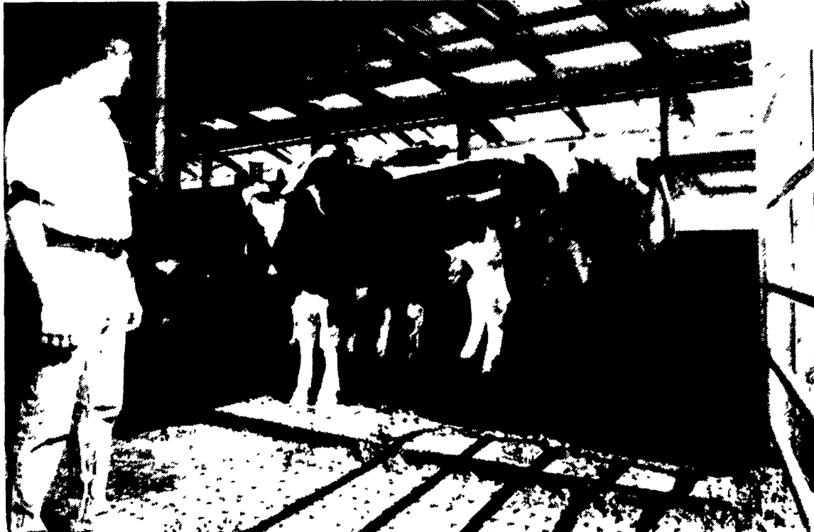
The slope of 2 inches per foot provides more of an angle for gravity and footwork to push the manure through slats, down eight feet. After the pit fills, a valve is opened and, in minutes, gravity pushes the manure into the huge manure pit outside.
