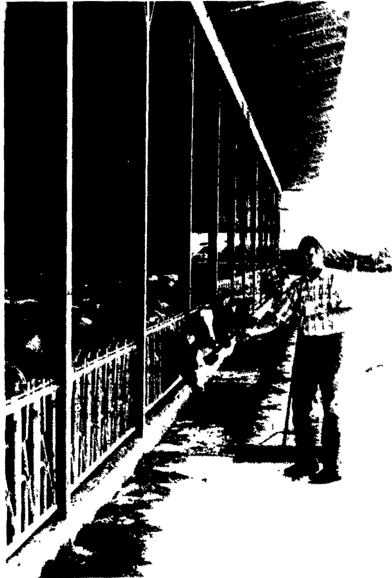
In the summer, the roof overhangs enough to prevent sun from heating up the 285 foot long heifer facility. There are seven heifers to a pen — they are placed in the first pen at one day old and are rotated up the other pens until they are two years old. Then, they are moved to the main freestalls.
