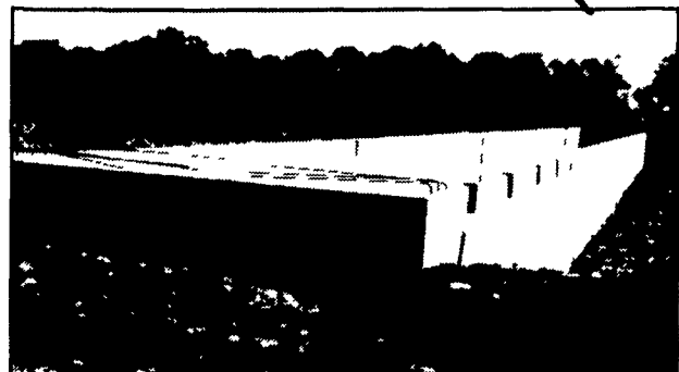
300' Long Manure Pit For Hog Confinement
