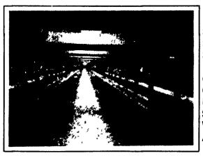
Standard Girter System Includes 3-2"x12" Girters, **Double Post-To-**Girter Bracing, Concrete Curbs Under Posts, And Steel Beams With Steel Posts At Pit Doors.
