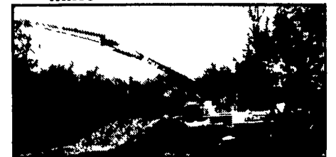
92' Boom Placing Concrete
