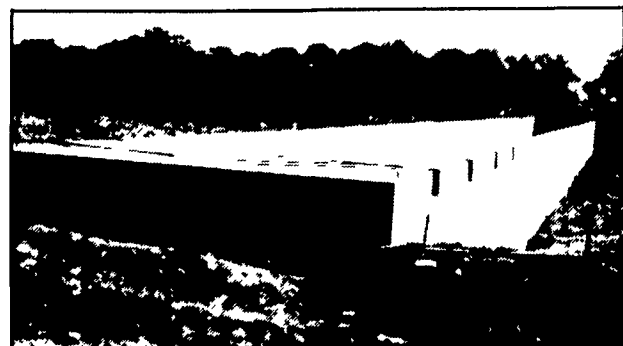
300' Long Manure Pit For Hog Confinement
