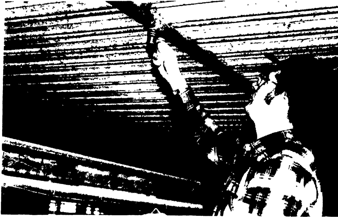
William Arble, technical specialist with PennTAP, checks out a sprinkler head at the Shenk farm. If a fire is detected, the sprinkler will activate for 20 to 25 minutes to help control and contain a fire.
