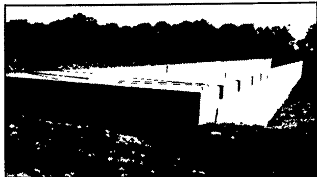
300' Long Manure Pit For Hog Confinement
