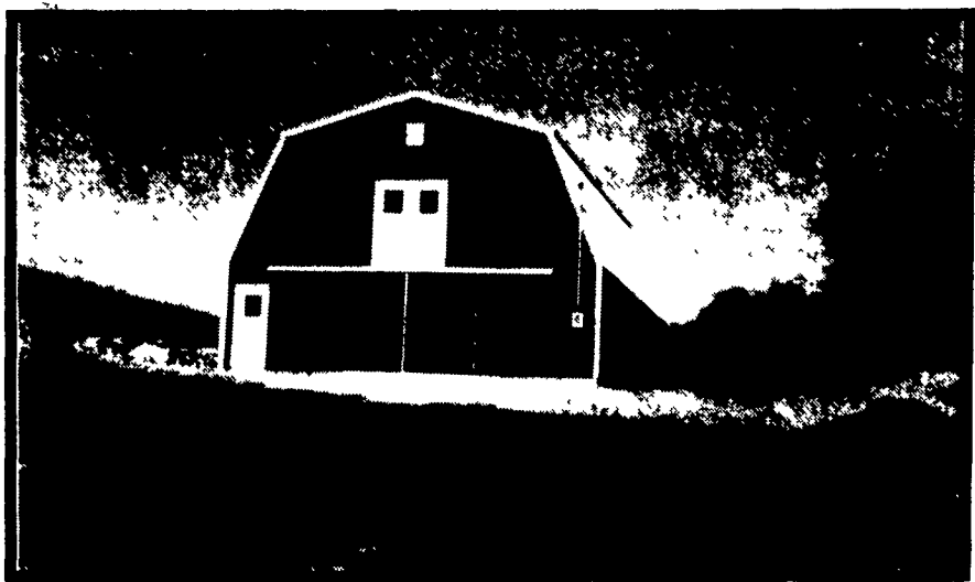
36'x48' Shed, featuring Gambrel Attic Trusses and Fabral Grandrib 3 Painted Steel
