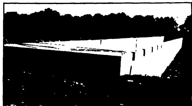
300' Long Manure Pit For Hog Confinement
