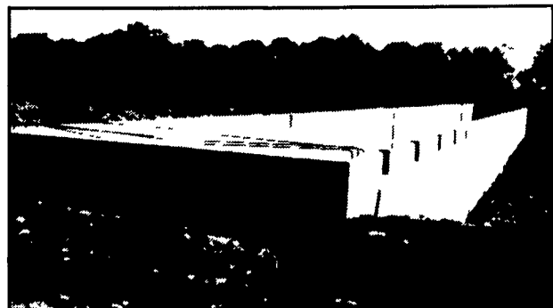
300' Long Manure Pit For Hog Confinement
