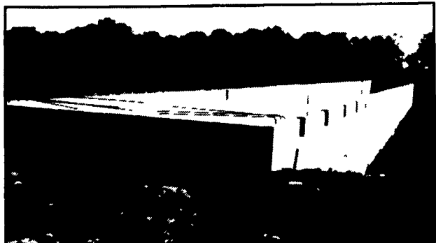
300' Long Manure Pit For Hog Confinement
