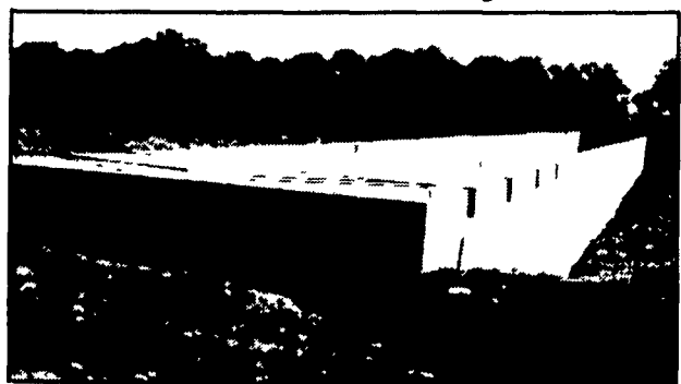
300' Long Manure Pit For Hog Confinement
