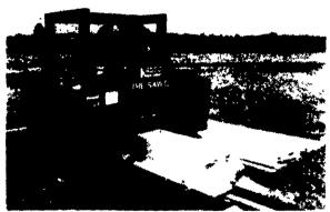
"The Saw II" is a band saw mill built to cut dimensional lumber from a log, accurately and smoothly The Kasco mill is built durable, having heavy 2"x3" tubing, 4" channel iron, and 1/4 "x10" plate in mill frame Track is of 4"x4"x½" angle iron Heavy shafts on which the blade wheels run are 1½" diameter and 37%" long, supported on each end with heavy ball bearings, giving extra stability and longer trouble-free life
