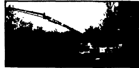
92' Boom Placing Concrete
