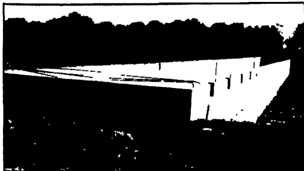
300' Long Manure Pit For Hog Confinement
