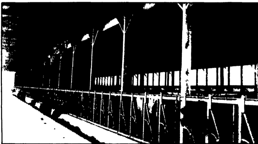
Pole Type Building With 32 Lb. Load Certified Trusses. All #2 Or Better Type Lumber.
