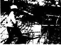
**S&S Silo Service** prepares the silo surface by using a 3,000 lb. pressure washer, thus making the silo moist, making a much better surface to bond
