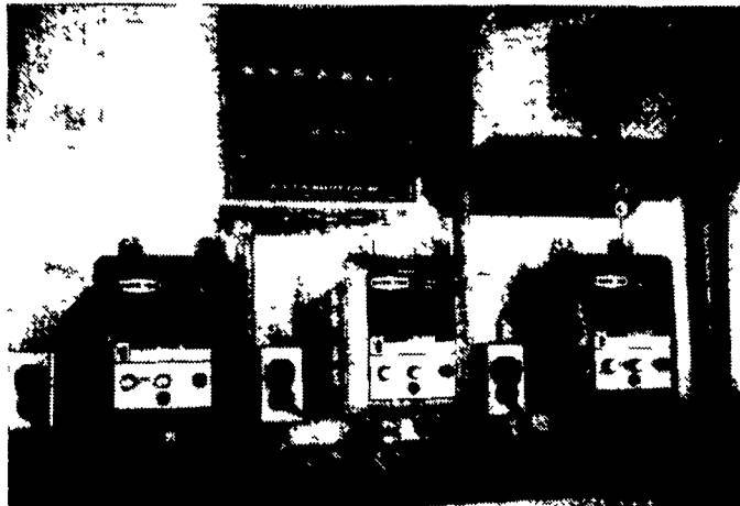
CHORE-TIME Electronic Fan Controllers With Temperature Read-Out And Variable Speed Controller For Collectors
