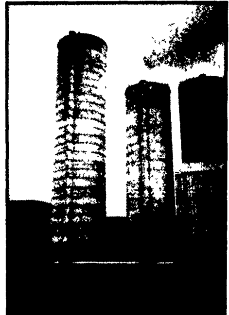
24'x104' Silo with Big Jim holds over 1600 tons corn silage.
